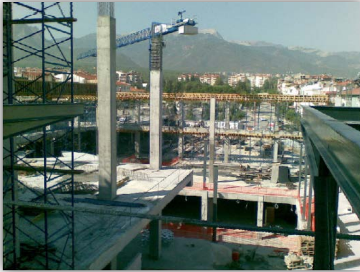
Figure 2. A View from Reference Construction Site Denizli, Turkey
