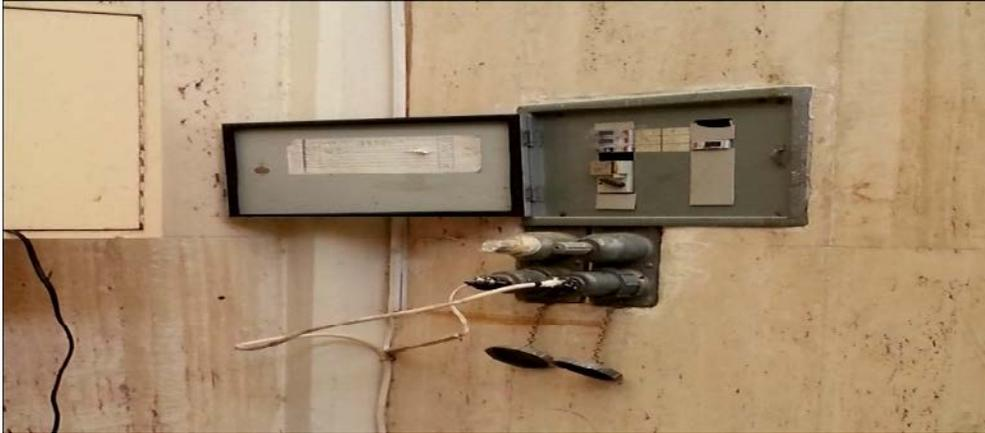
Figure- 17(c): Exposed electrical box in KCBB.
