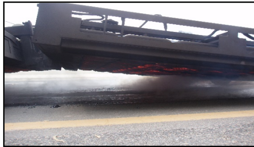
Figure- 5 Pre-heating unit
