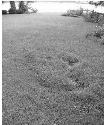
Figure 2. Failing septic system on north end of Hilton Head Island with Intracoastal Waterway in background.
