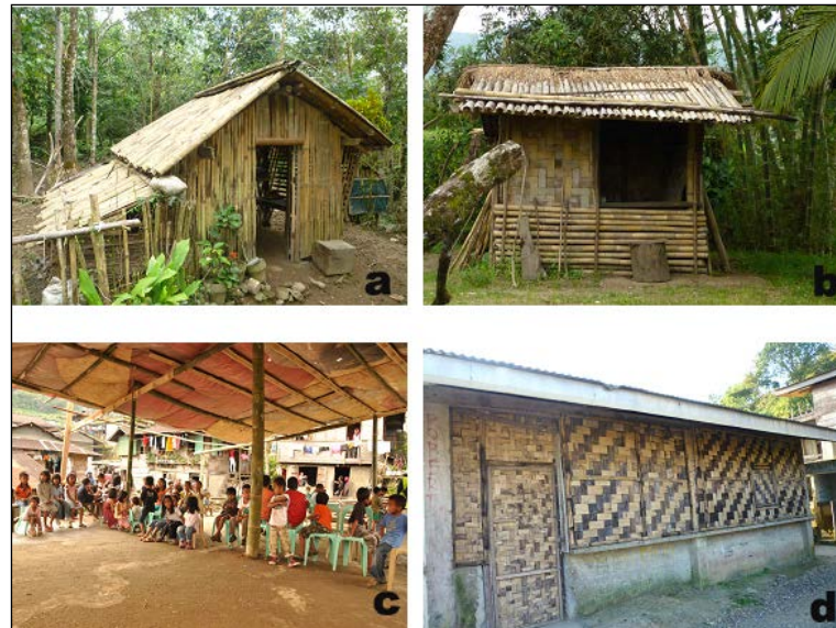
Figure 7. Byuyu as house construction materials; sigey (a), teyob (b), byawi (c) and bulilaw (d)
