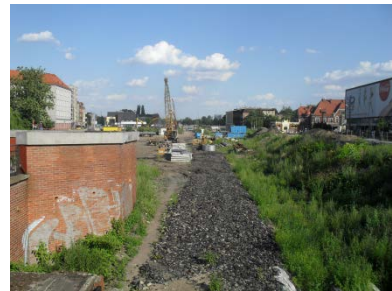
Fig.7. View - east side
