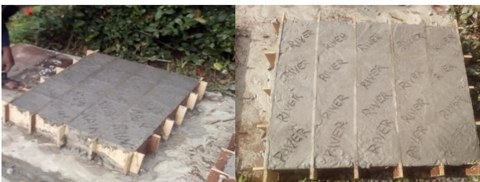
Plate 2: Concrete compacted in formwork and labelled
