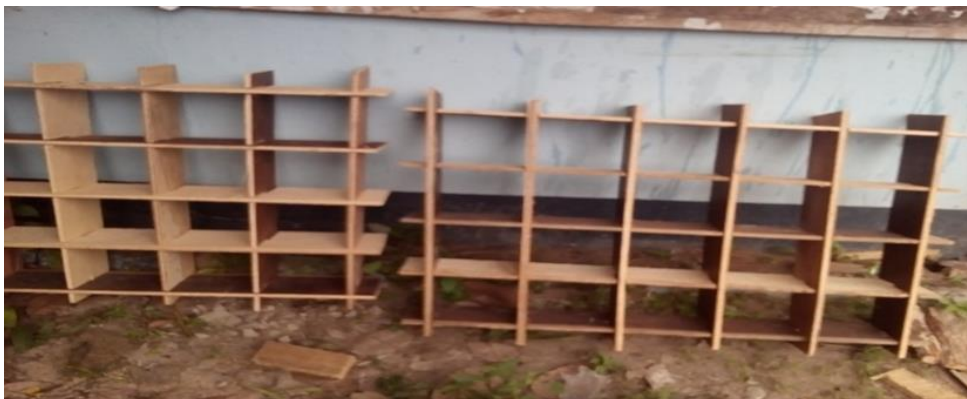
Plate 1: Completed formwork to receive concrete
